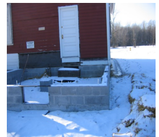
Foundation for Schoolhouse addition
